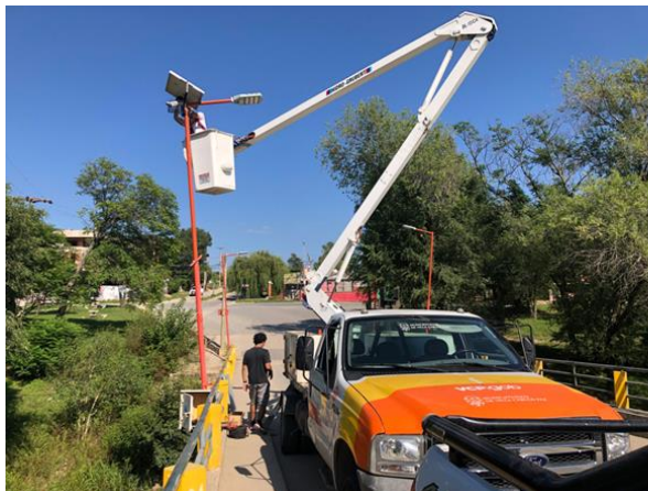
Figure 8: LSPIV Station installed in Villa Carlos Paz, Córdoba (left) and view of installed equipment (right)
