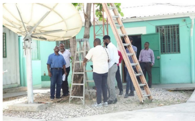
Figure 23. Enhancing data access: GEONETCast system installation in Haiti
